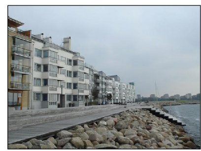
Coastal Rocks As Engineers spec
