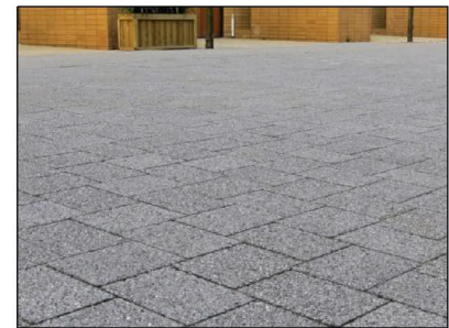
Proposed Concrete Paving Blocks
