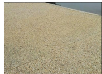
Proposed Exposed Aggregate Paving
